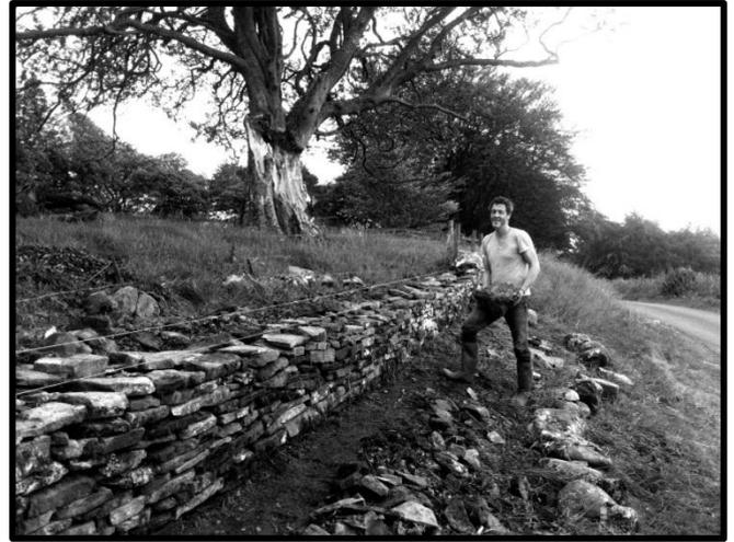
*Tying a line of string from one end of the broken wall to the other, I organised the wall rubble into piles and slowly started re-building, with large rocks to the outside of the wall and small stones in the middle, to create an interlocking formation. With the craftsmanship of the existing wall evident, it was a privilege to make my own contribution – hopefully it, too, will stand the test of time!*
